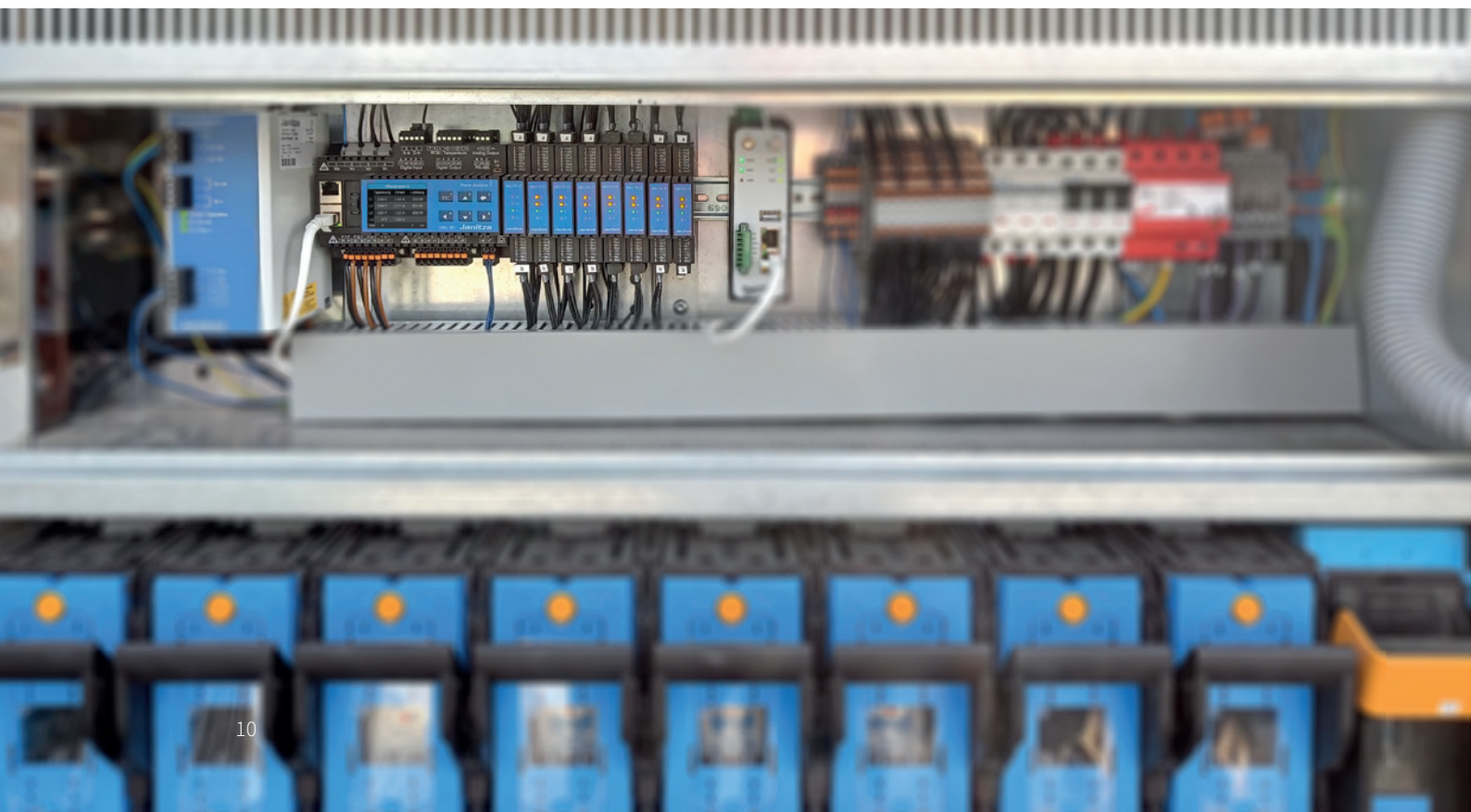
UMG 801 with modules in a secondary substation
