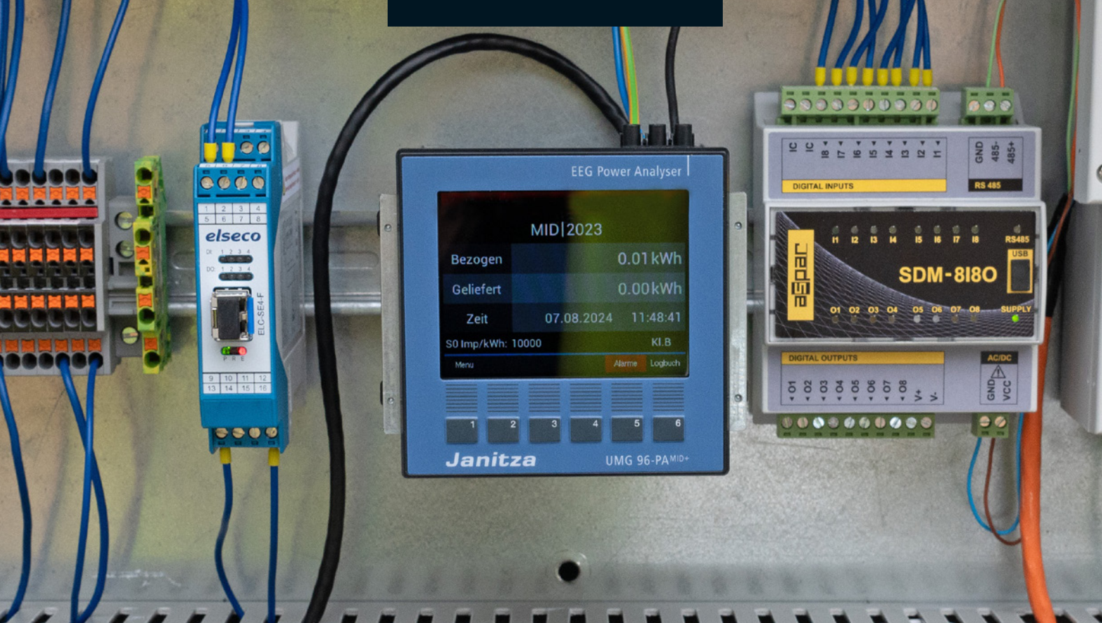
The MID-certified UMG 96-PA-MID+ records legally compliant measured values in the PV park's transformer station (in accordance with Directive 2014/32/EU)
