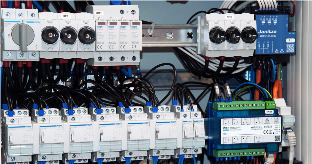
The UMG 103-CBM universal measurement device on the top right enables precise determination of the PUE value
