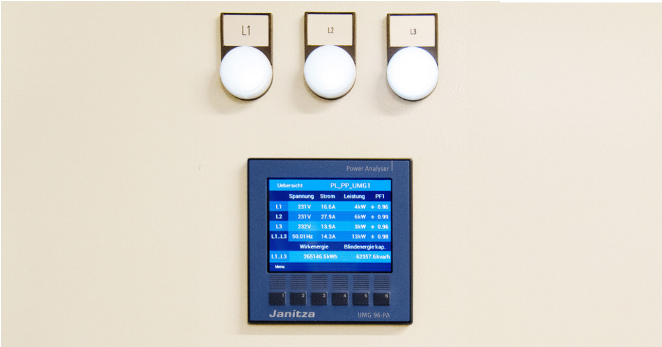
UMG 96-PA power analyzers from Janitza replace the old door-mounted devices
