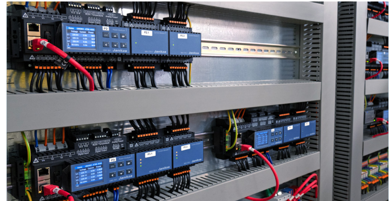
The expandable modular power analyzer UMG 801 can be expanded with modules
