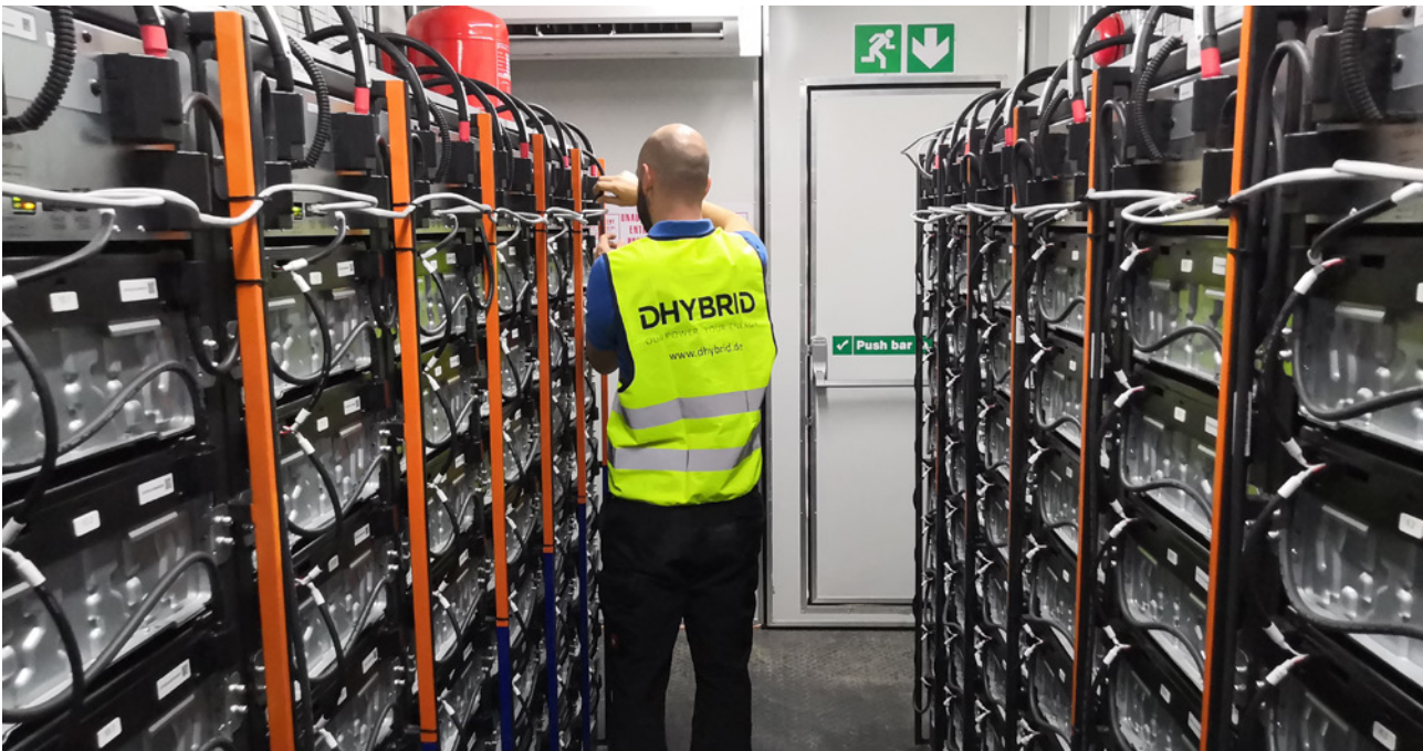
With a capacity of 1,027 kWh, the lithium-ion memory units bridge the nights and days with little sunshine
