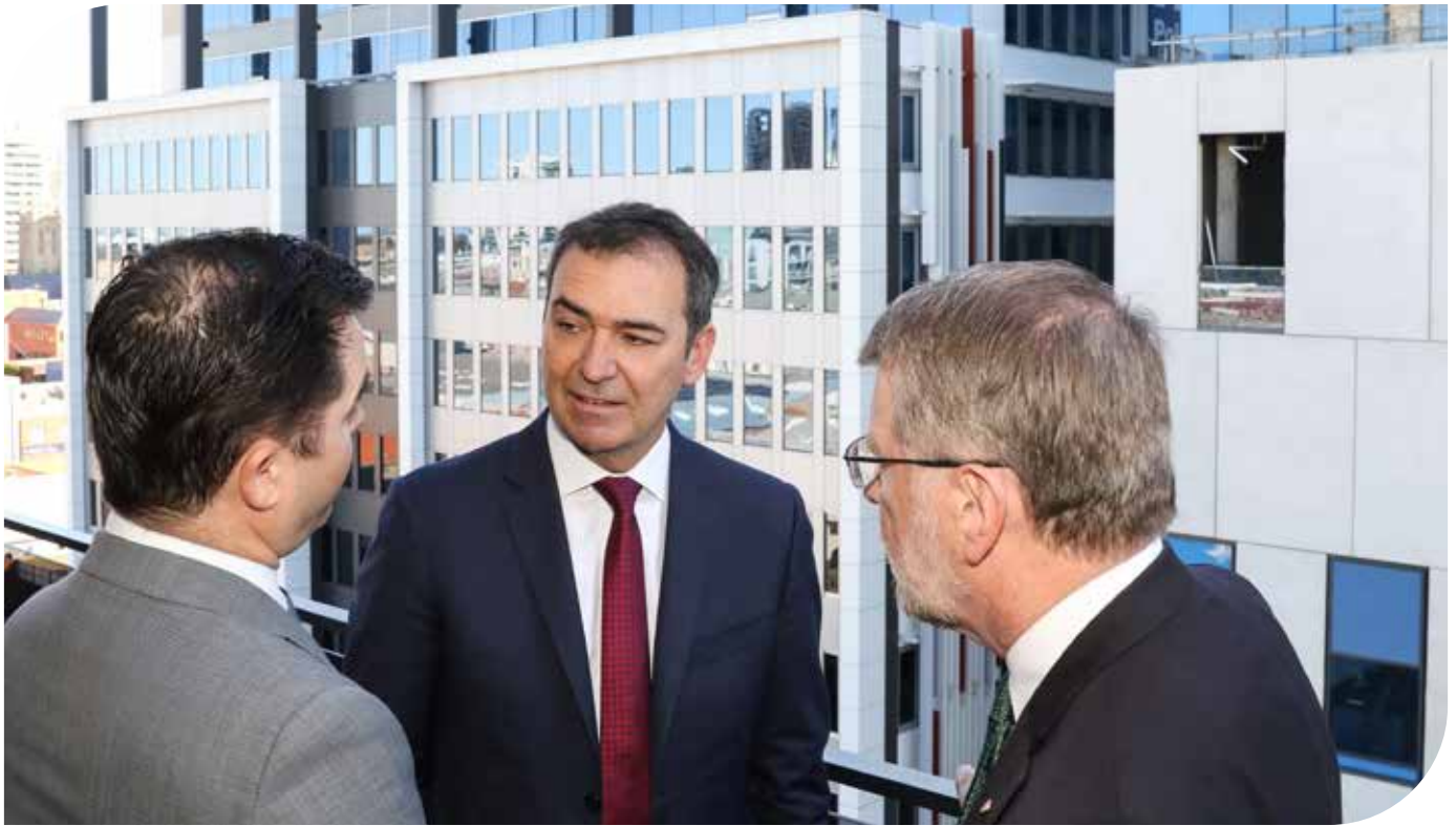
On 14 August 2018, (L-R) Commercial and General Executive Chairman Jamie McClurg, SA Premier Steven Marshall and Calvary Chair John Watkins AM attended an important 'topping out' milestone of Calvary Adelaide Hospital construction at 12 storeys high.
