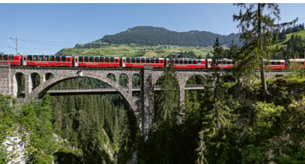
3 Solis Viaduct/Solis, 863 m a.s.l.
