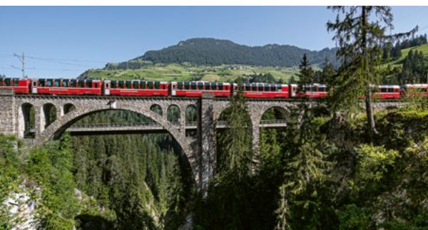
3 Solis Viaduct/Solis, 863 m a.s.l.
