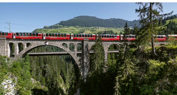
3 Solis Viaduct/Solis, 863 m a.s.l.
