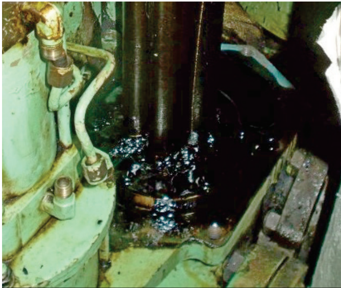
Fuel filter – visible heavy sludge, which blocked the filter completely
