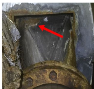
Cracks on water drain outlet (viewed from outside) with signs of leakage
