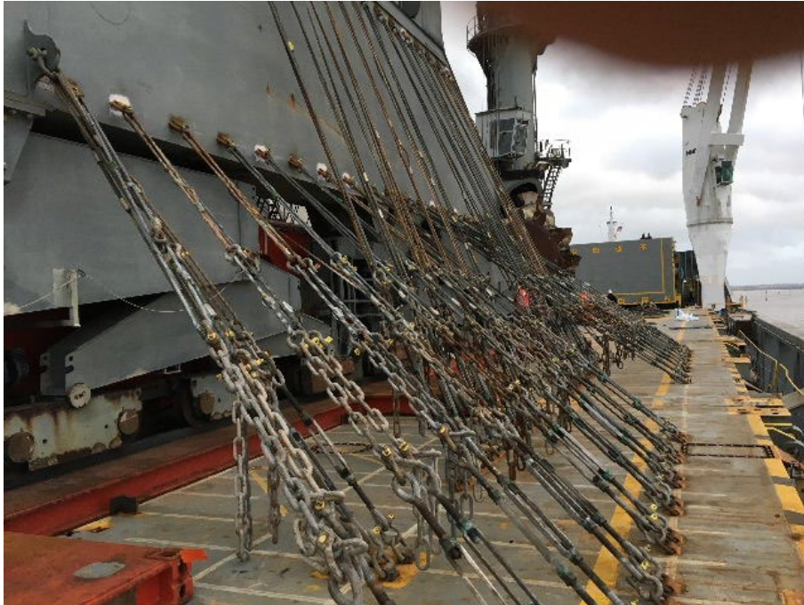
A closer view of steel wires, chains and turnbuckles securing project cargo to the ship's deck
