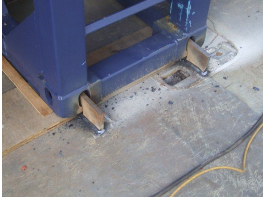
Steel stoppers welded to the deck and securing purposely made frames supporting project cargo Note anti-slid plywood boards placed underneath the blue frame
