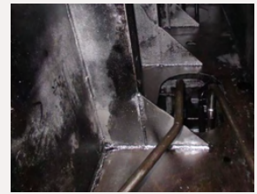
Bunker tank cleaned after debunkering fuel with high catfines
