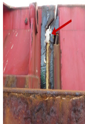
Foam between hatch covers
